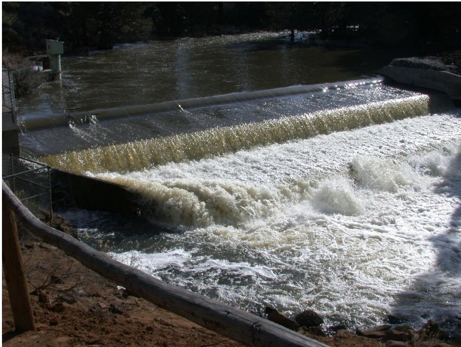
Figure 2. Velocity barrier operating on Pine Creek during spring snowmelt.
